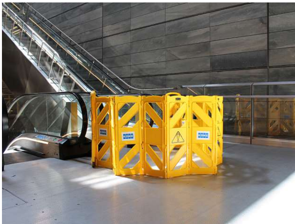
Figure 131: Escalator during maintenance
