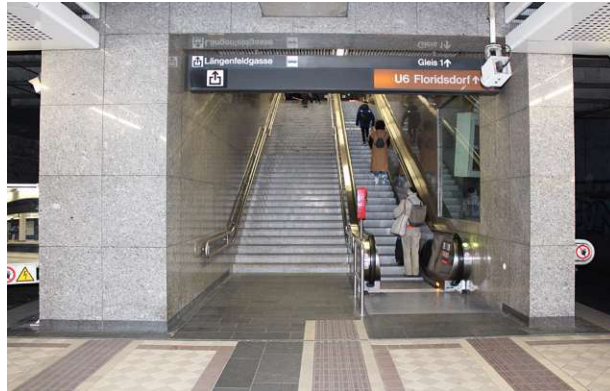
Figure 115: Exemplary exit without elevator at Längenfeldgasse station
