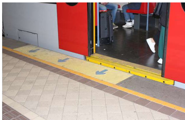
Figure 117: Floor markings U6 on platform 2
