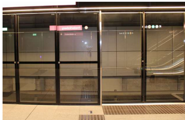
Figure 18: Glass portals on platform M3
