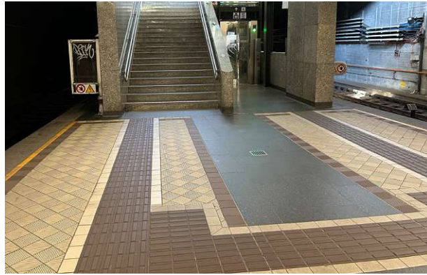
Figure 91: TWSIs led to the left handrail from platform level
