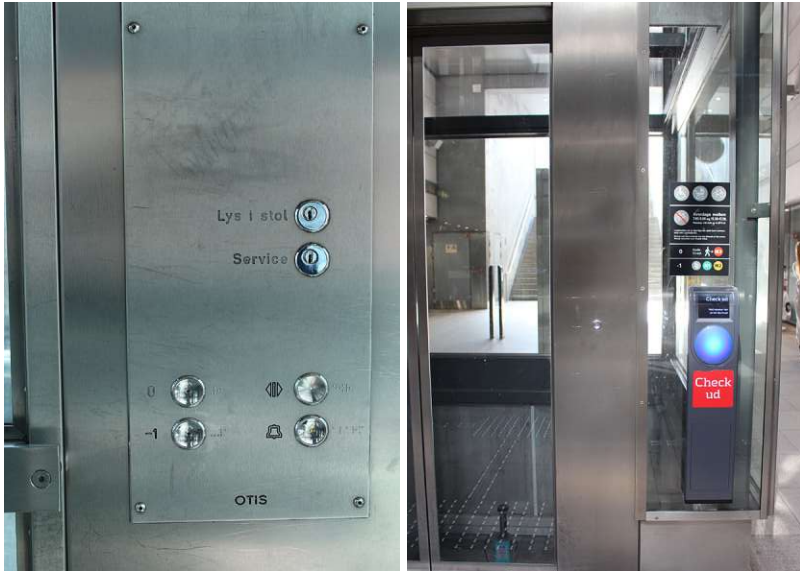
Figure 143: Operating elements E2 inside and E1 outside
