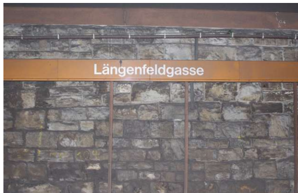
Figure 116: Signage on the wall opposite the platform
