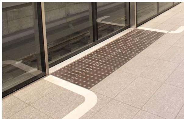
Figure 34: Floor markings on platform M3
