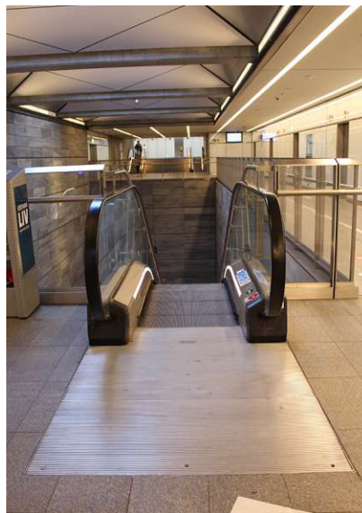
Figure 77: Exemplary ribbed metal surface in front of escalators
