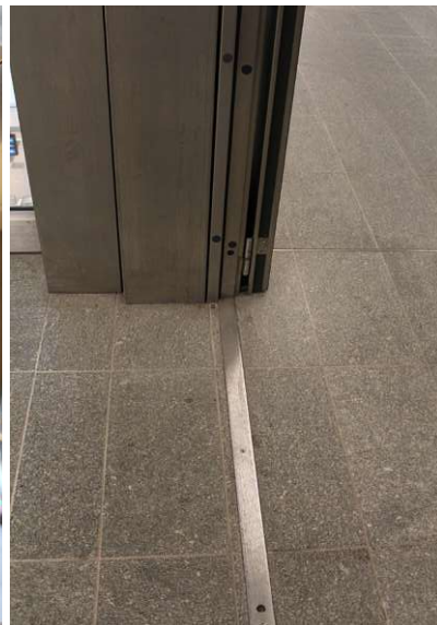
Figure 129: Door frame on passage level
