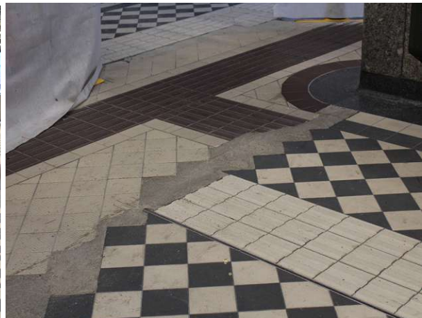
Figure 158: Entrance building 2 detail construction work
