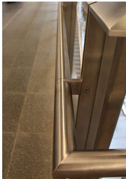
Figure 81: Handrail on passage level
