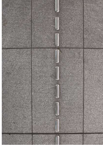
Figure 74: TWSIs in the older part of the station
