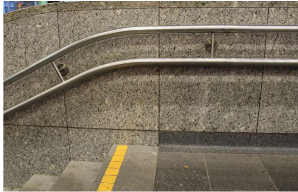
Figure 101: Double handrail for stairs
