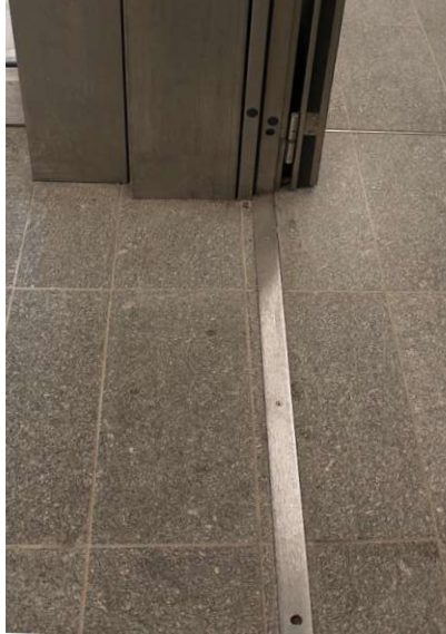
Figure 80: Door frame on the ground
