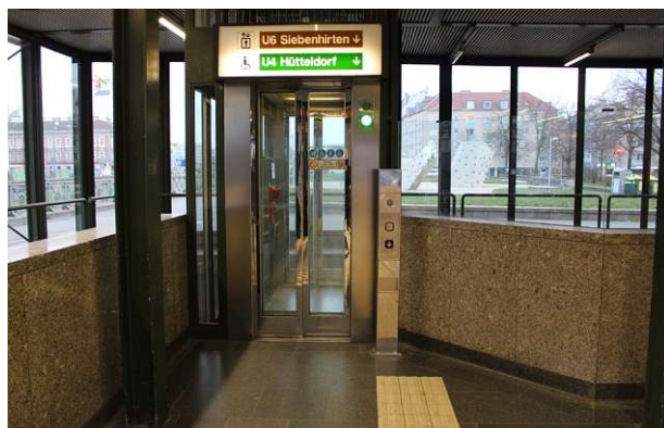
Figure 93: Operating buttons of the elevator on a separate pillar
