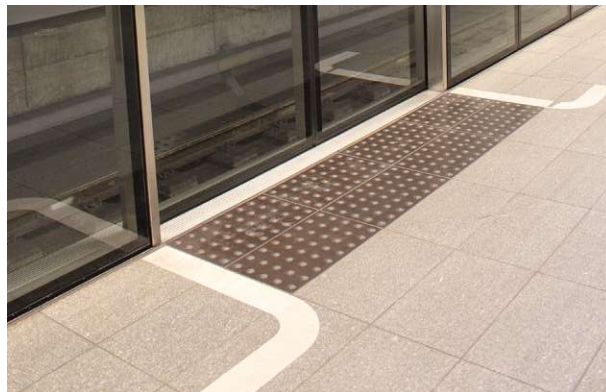
Figure 46: Floor markings on platform M3
