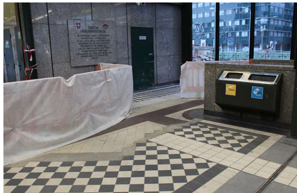
Figure 108: Construction work in the entrance area
