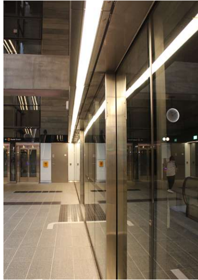
Figure 85: Lighting next to entrance doors on platform M3
