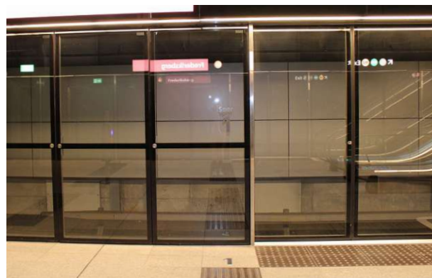
Figure 58: Glass doors on platform M3
