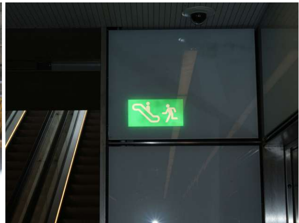
Figure 132: Escalator as emergency exit
