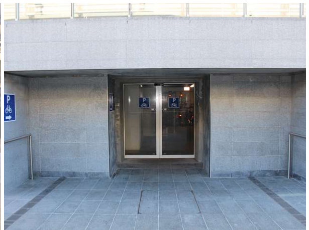
Figure 125: Glass door on entrance level
