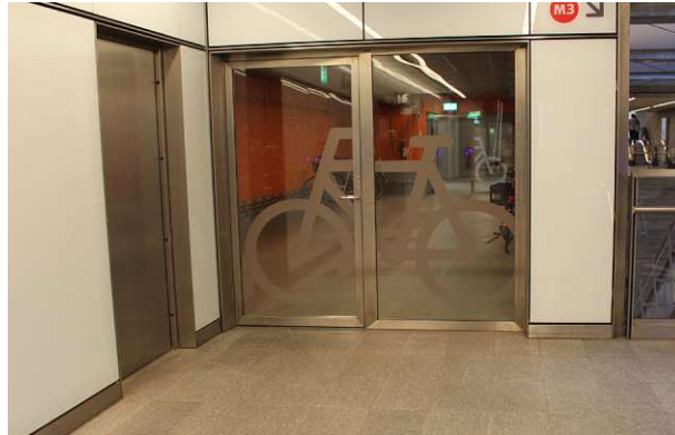
Figure 38: Door marking on passage level
