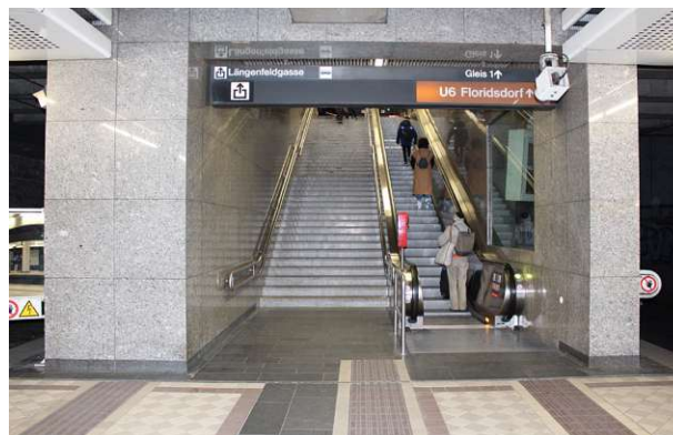
Figure 98: Connection between TWSIs and escalator
