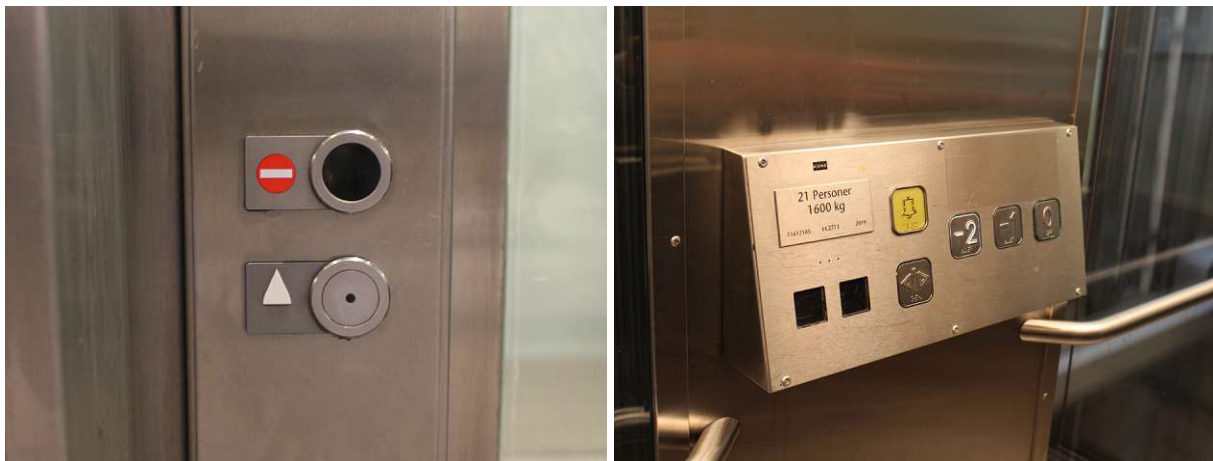
Figure 55: Operating elements inside and outside E3 and E4
