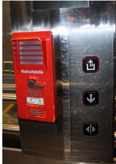
Figure 107: Operating elements inside E5
