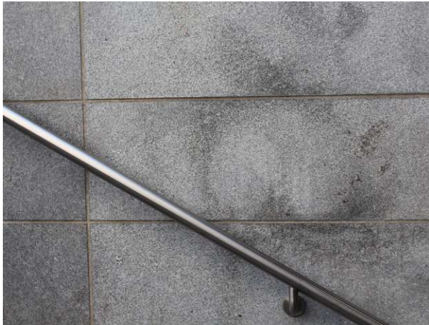
Figure 126: Handrail on entrance level
