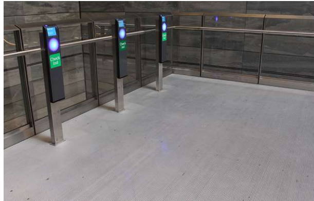
Figure 82: Intermediate level of escalators led to platform M3
