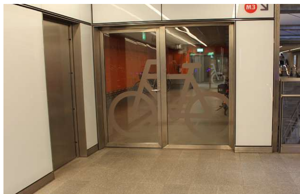
Figure 64: Door marking on passage level
