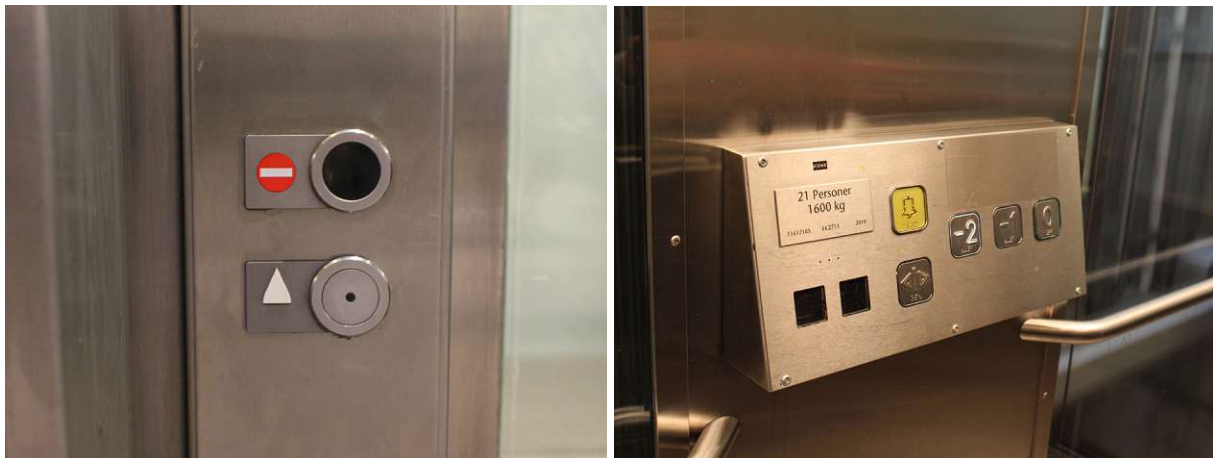
Figure 39: Operating elements inside and outside E3 and E4
