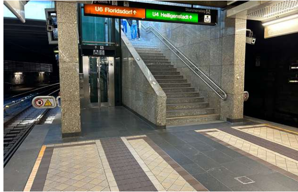
Figure 94: Criticized distance from the middle wall to TWSIs
