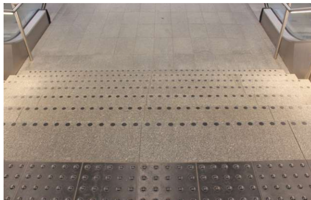
Figure 22: Stair marking on passage level
