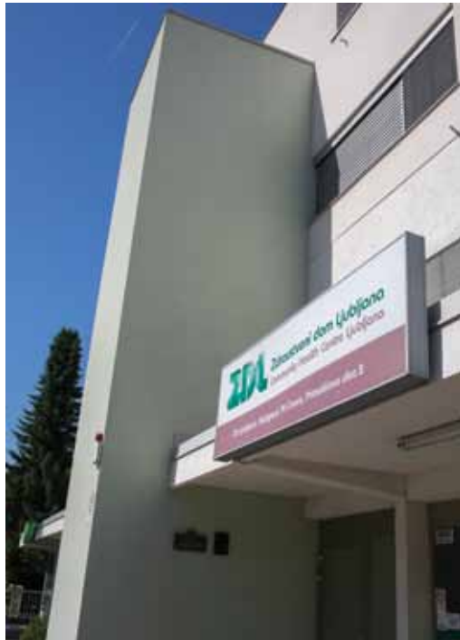
A built-in lift at the Ljubljana Health Centre unit in Črnuče (photo: Miha Fras)
