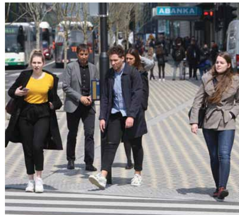
Dropped kerb access and protruded grip floor warning markings at pedestrian crossings (photo: Nik Rovani)
