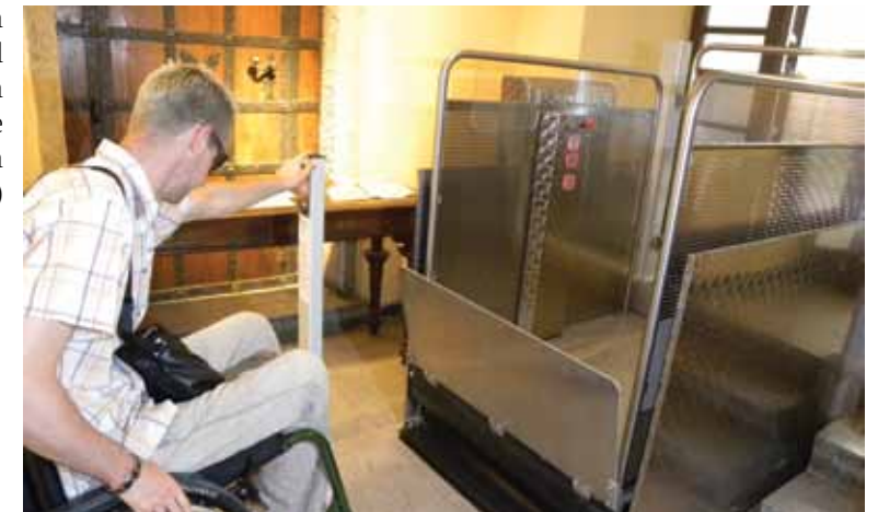
Lifting platform in City Hall (source: Association of Paraplegics of the Ljubljana Region archive)
