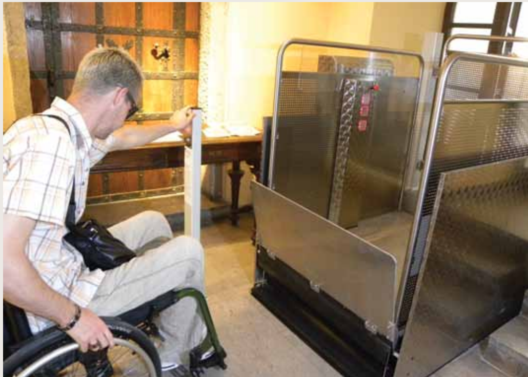
Lifting platform at the City Hall, photo: Association of Paraplegics of the Ljubljana Region archive
