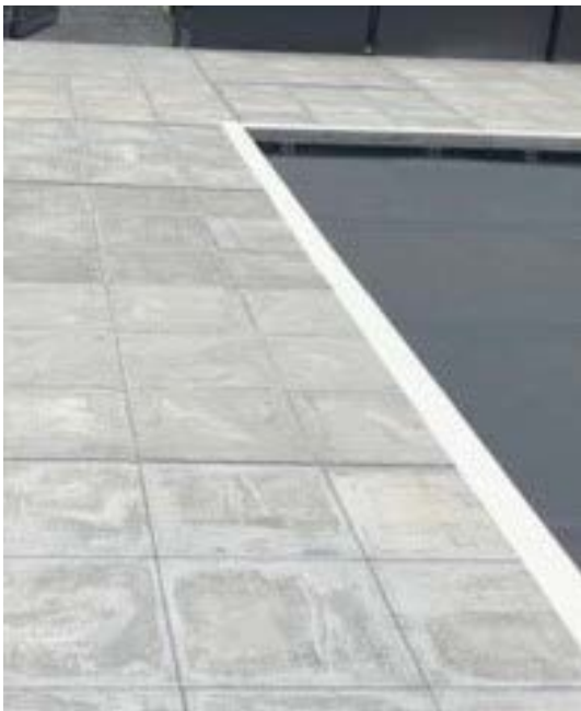
Figure 13 – Photo of the simulation of a segregated cycle-footway with a white kerb upstand delineating both sides. The surface for pedestrians is grey pavement and black tarmac for cyclists.
