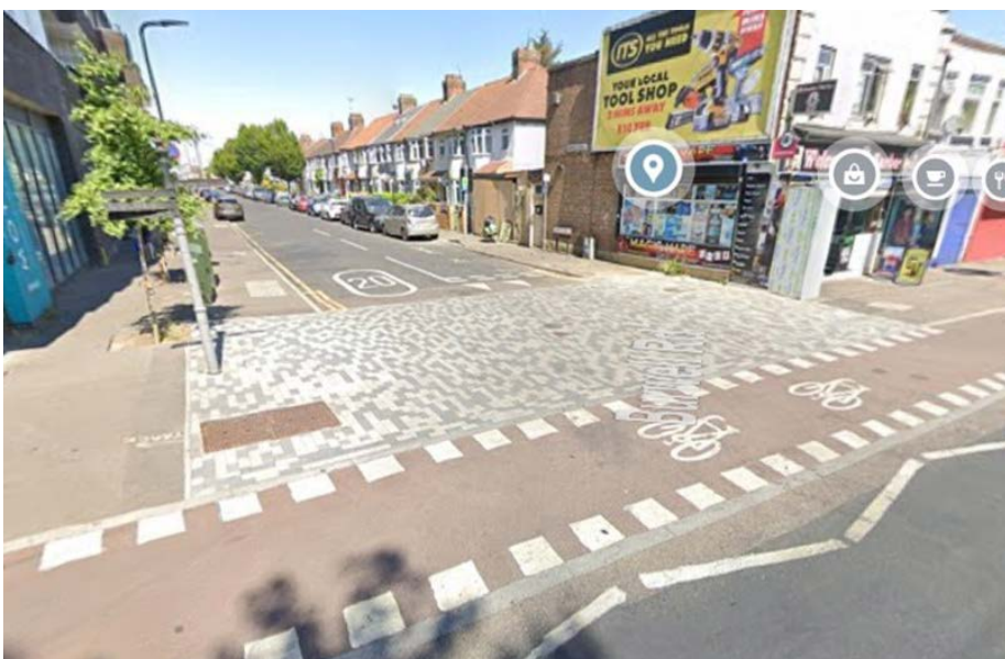
Figure 9 - Lea Bridge Rd and Burwell Rd Junction, a continuous footway setup where the raised pavement uses white-grey pavers, the footway and cycling lane are of a reddish hue. The setup has no obvious clutter.
