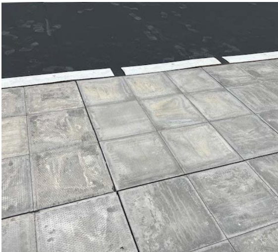
Figure 12 - Photo of the simulation of a segregated cycle-footway with a white trapezoidal delineator with gaps. The surface for pedestrians is grey pavement and black tarmac for cyclists.
