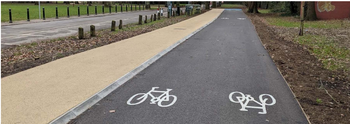
Figure 6 - A segregated cycle-footway with buff coloured surface on the pedestrian side and black asphalt on the cycle path with a low kerb delineator running down the middle of the path. (Source: Welsh Government (2021) Active Travel Act Guidance, https://www.gov.wales/active-travel-act-guidance , accessed 18 July 2024).
