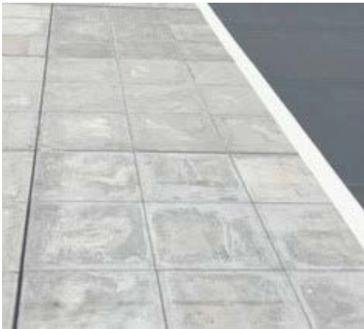
Figure 14 - Photo of the simulation of a segregated cycle-footway with a painted white line used as the delineator. The surface for pedestrians is grey pavement and black tarmac for cyclists.
