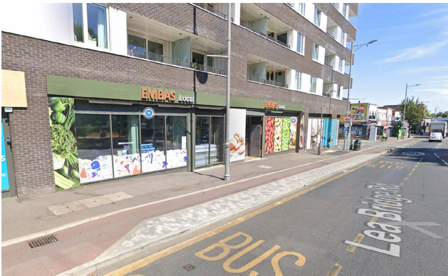
Figure 8 - A Shared Boarder Bus Stop (SBSB), Stop LE, with a buffer area demarcated by white-grey pavers covering approximately 1 meter. The cycling way and footway have a similar colour (red-ish hue). There is some clutter around the flag, a streetlamp, a rubbish bin, and one pole and bollard with no apparent function. There is no tactile paving indicating the transitioning from footway to cycling lane, instead a forgiving kerb is used.
